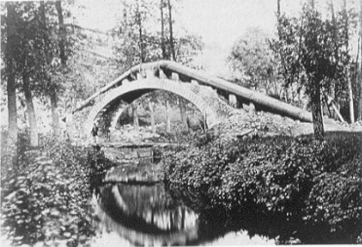
99. Hippolyte Collard, Pont de Chézy (Aisne) — State of the Project on October 3, 1864 , from Dérivations des sources de la Dhuis , n.d.
